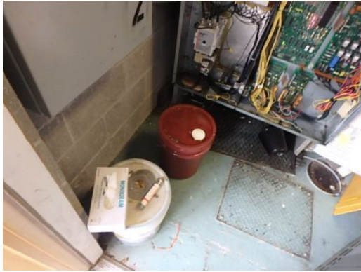
#19 ELEVATOR MACHINE ROOM
