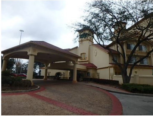
#1 FRONT (SOUTHWEST) ELEVATION
