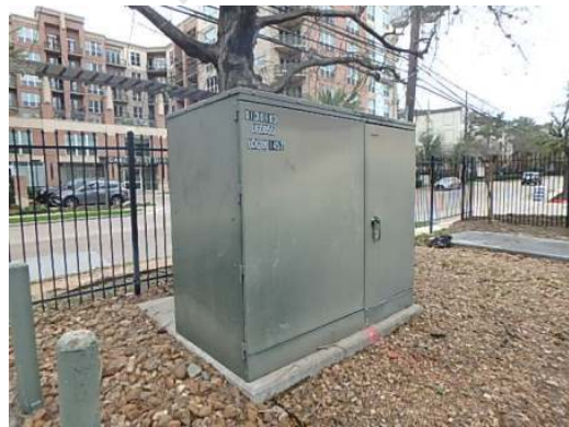
#18 PAD-MOUNTED TRANSFORMER
