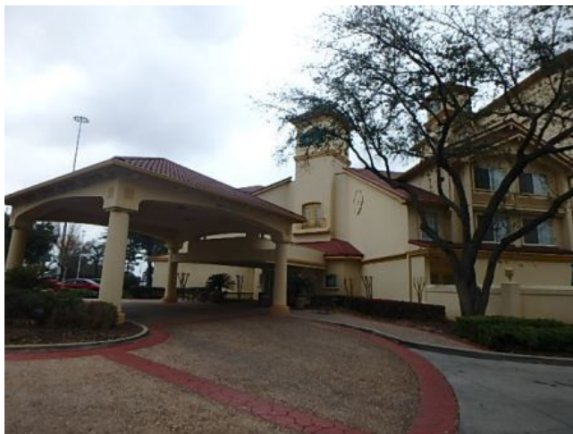
Front (southwest) elevation
