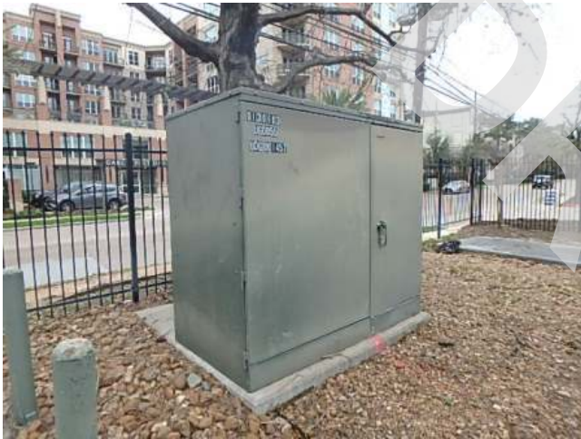
Pad-mounted transformer
